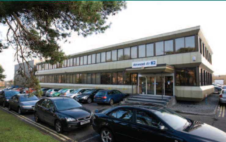
Advanced Air UK factory and technical centre of just over 60,000 sq ft
